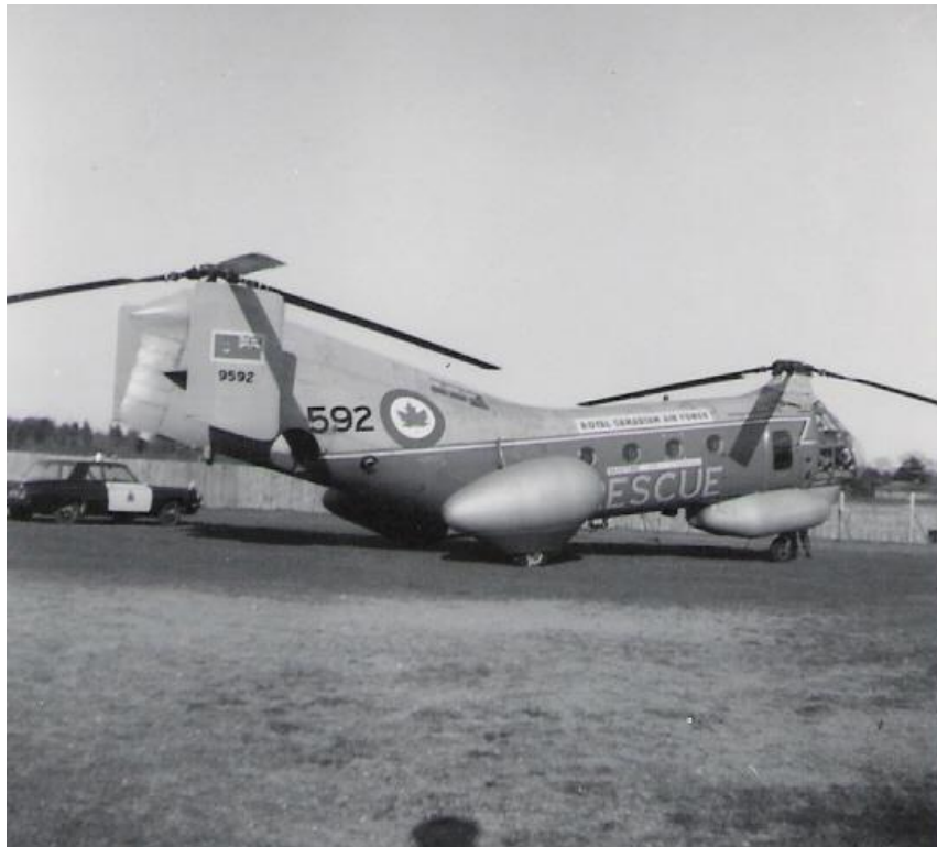
Three different floatation systems were tried, some for water operations and others for snow. The systems, when activated, inflated rubberized air bladders, thereby keeping the helicopter upright and afloat. The early systems were unwieldy, caused aerodynamic drag, and were unstable on anything other than flat, calm water. Shown is Vertol H-44A 9592 in Liverpool, Nova Scotia, sporting the third and best system developed, the low-drag floatation system. (Note the similarity to the later Labrador sponsons)
