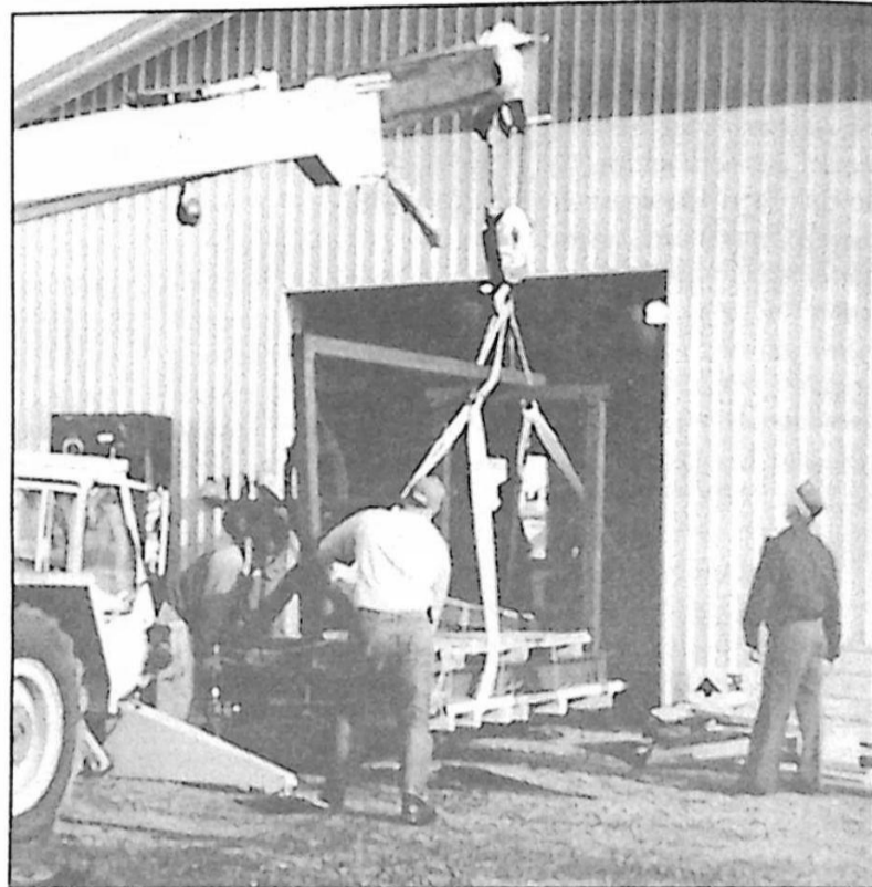
The Y2K Spitfire restoration project fuselage jig is carefully placed inside the Tet Walston hangar. The jig recently arrived from England and will be used for the construction of the Spitfire fuselage.
