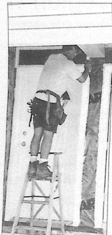
CE carpenter Dave Gallagher.
