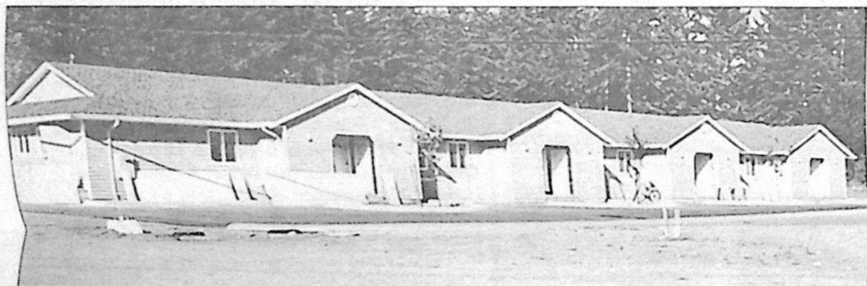
Almost completed single quarters unit, fourth of a planned five.
