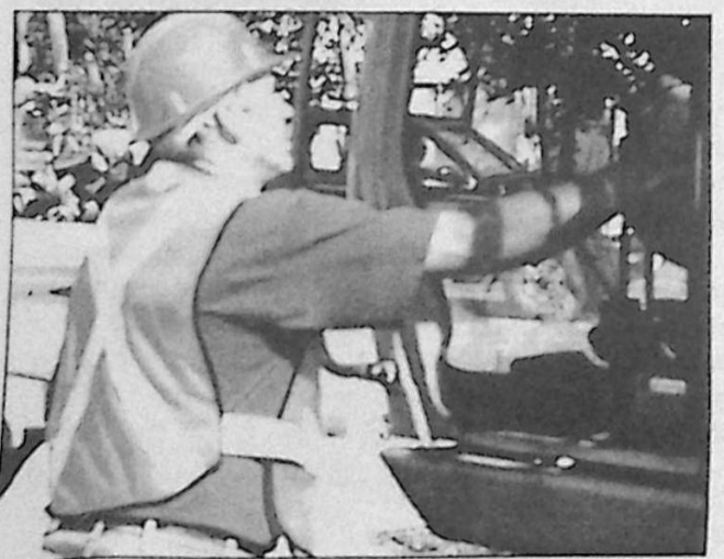
CE plumber Dan Dupuis confers with driver of large backhoe.
