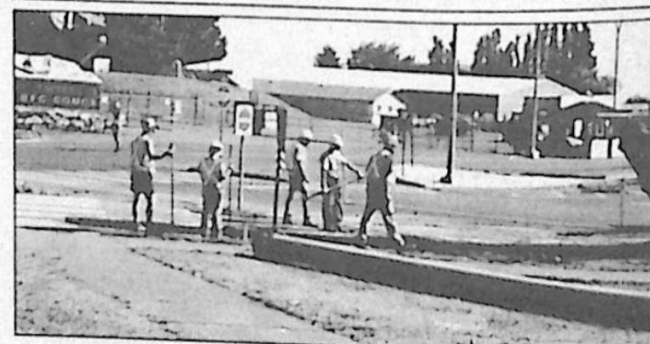
Airfield & Works crew with pipes ready to go in newly-dug trench.
