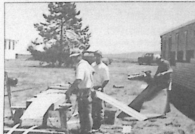
Members of CE's Structural Team at Quadra: Tom Woodman, Steve Darvaul and Lance Callerae prepare siding for the quarters...
