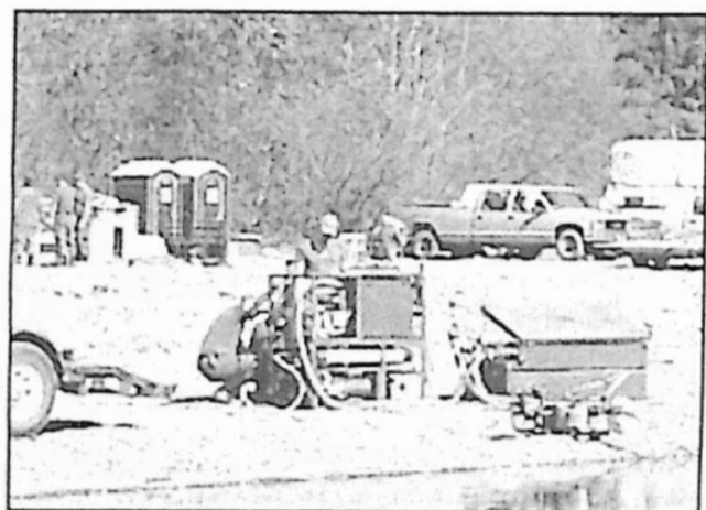
Water plant being set up.
