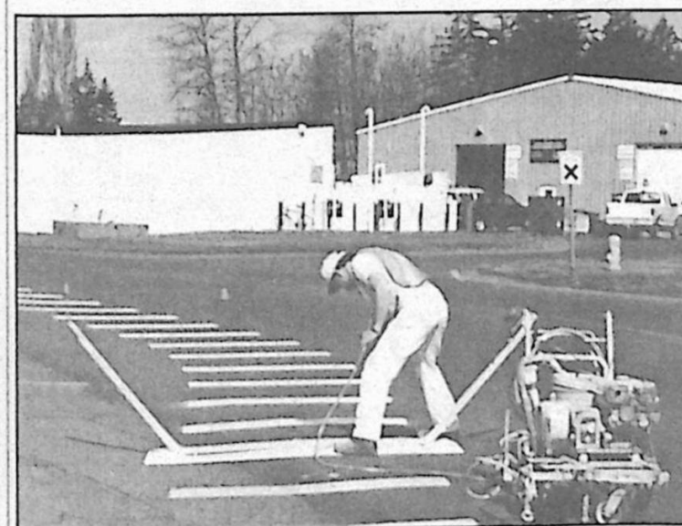
CE painter Glen Hendry freshening sidewalk lines.
