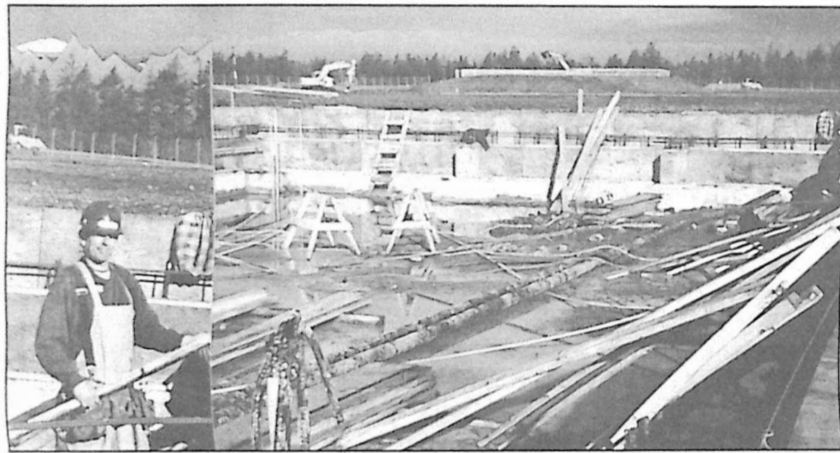
Working on foundation for the pre-fab office building on the Ammo Storage site.
