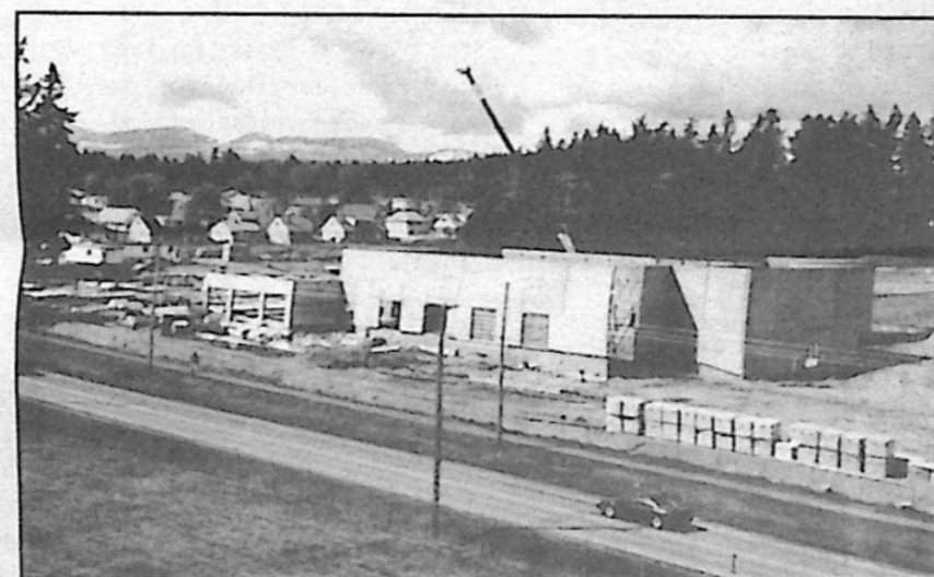
Beginning to see the shape of things to come.
