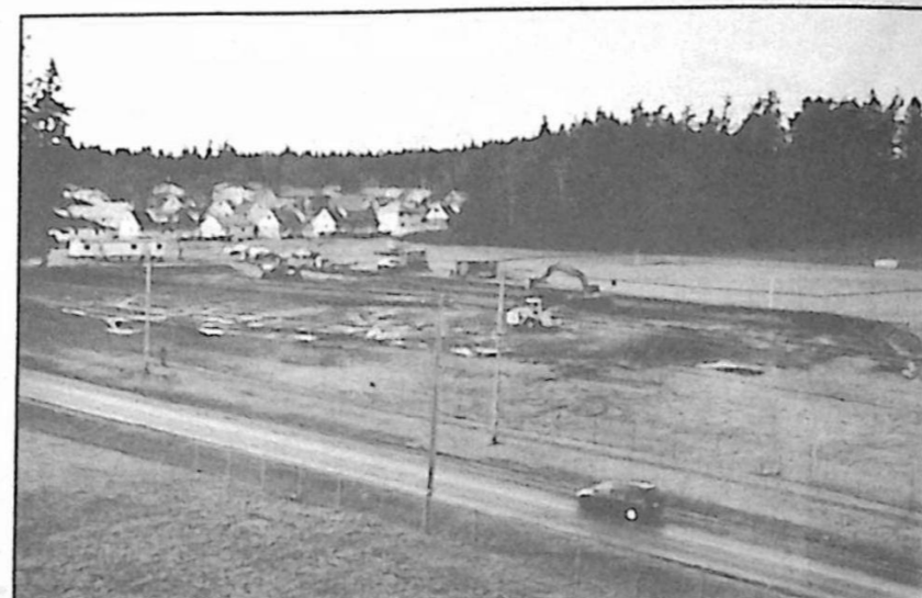
Just a hole in the ground.
