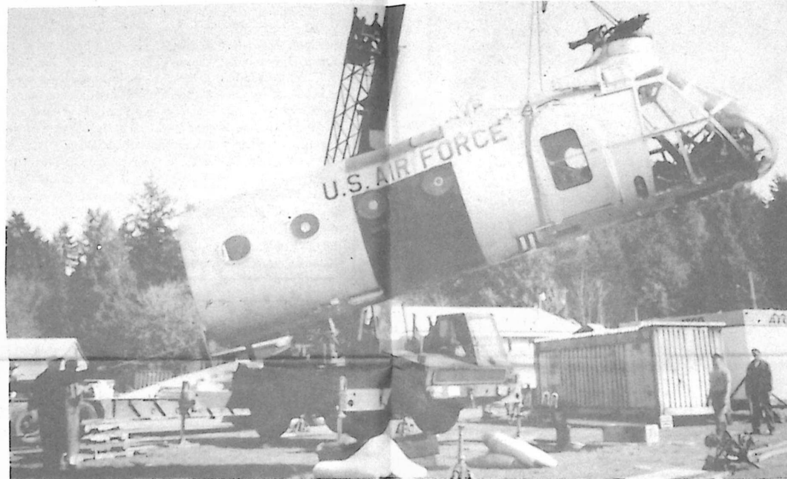
With the assistance of a heavy lift crane from CFB Chilliwack, the H-21 is lifted for placement on a transport truck.
