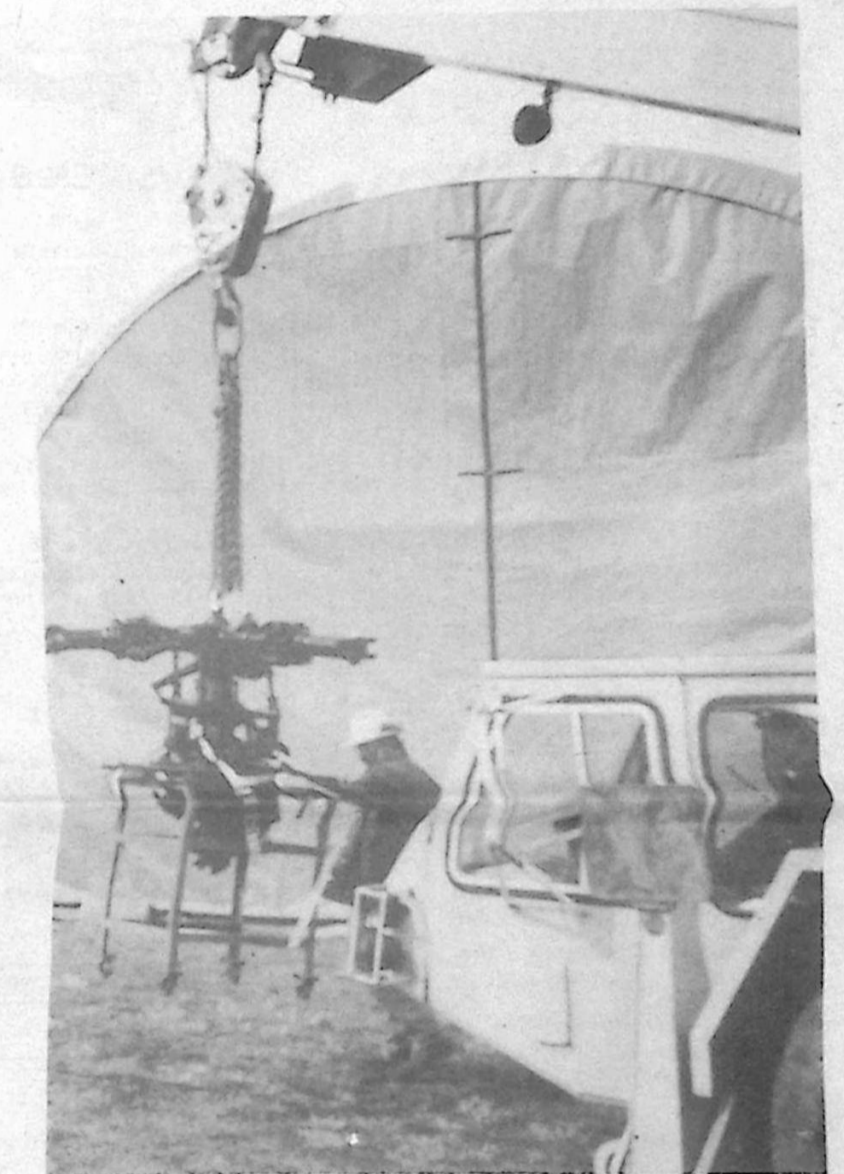
The restored rotor heads arrive for installation.
