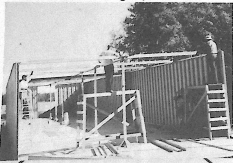
Assembling one of the auxiliary buildings for the Air Cadet Squadron.
