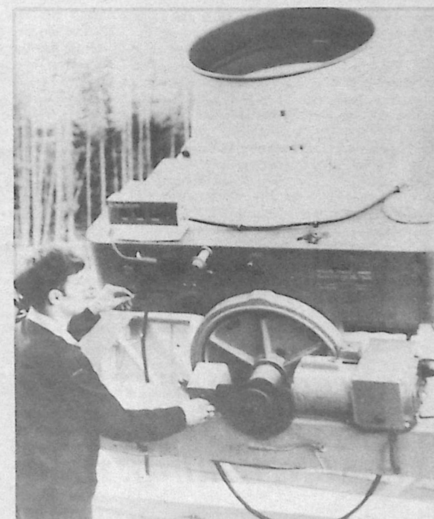
CANADA'S SPACE CAMERA -- Canada contributes one sensor to NORAD's space detection and tracking system. This Baker-Nunn camera at CFB Chatham, New Brunswick, is capable of photographing the light reflected from an object the size of a basketball fifty thousand miles in space.
