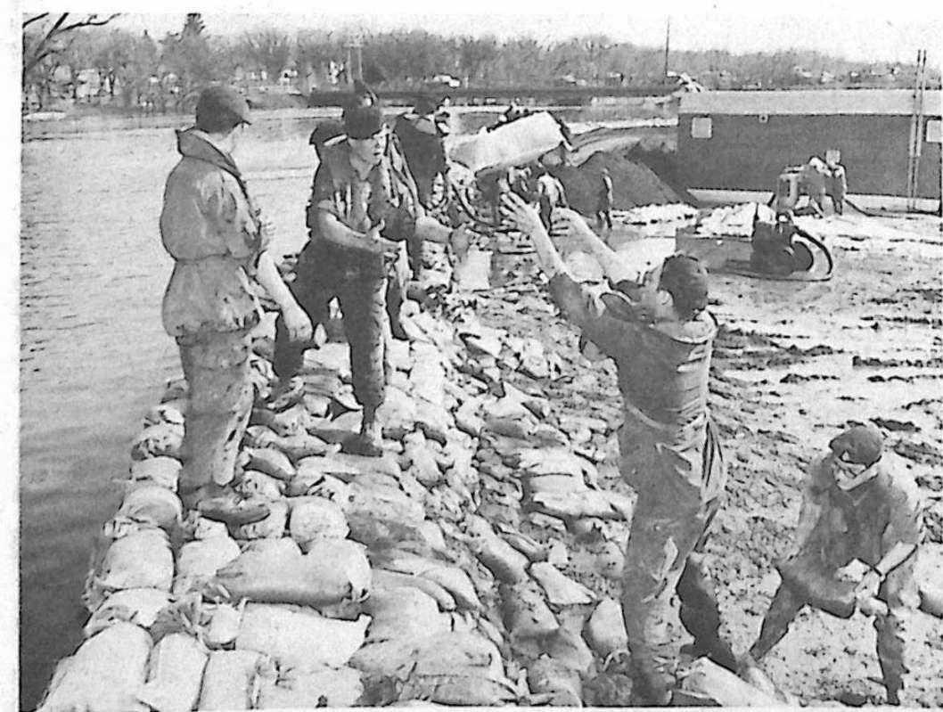
WINNIPEG -- Members of the 3rd Regiment Royal Canadian Horse Artillery, CFB Shilo construct a dike around the pumphouse at Souris, Man. when it was threatened by floodwaters on the Souris River recently. The water rose a record 16 feet and more than 100,000 sandbags were used in the operation. The gunners also assisted in saving a number of homes further down river at Wawanesa.
