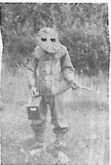
Nuclear Defenceman Cpl. F. P. Wilson wears a contamination suit especially designed to protect him against radioactivity. The Decontamination Control Meter he is holding is used in conjunction with the suit during the cleaning up period after fallout.
